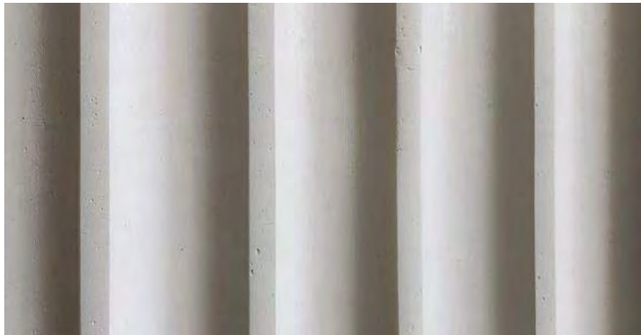
CONC1 FLUTED PRECAST CONCRETE
